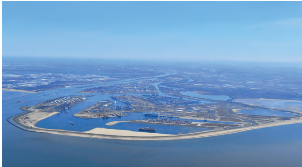
Rotterdam: recently completed the Maasvlakte Distribution Park West.
